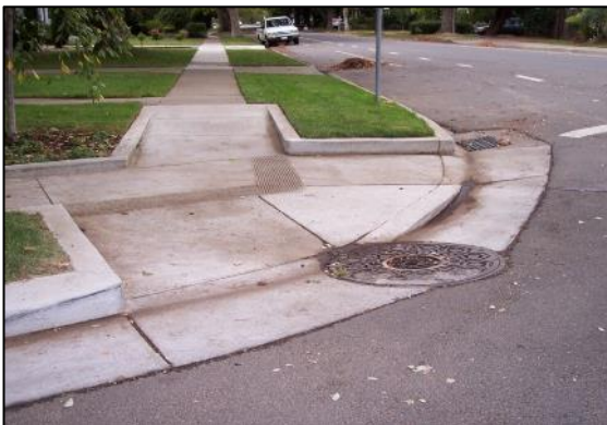
Example combination curb ramp, with a perpendicular ramp to a common landing and adjacent parallel ramps.
