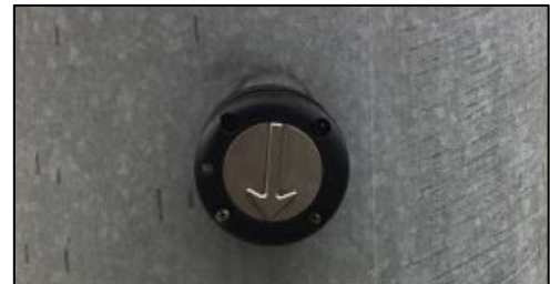
Example of pushbutton that is 2" diameter and includes tactile directional arrow on the pushbutton but arrow points down.
