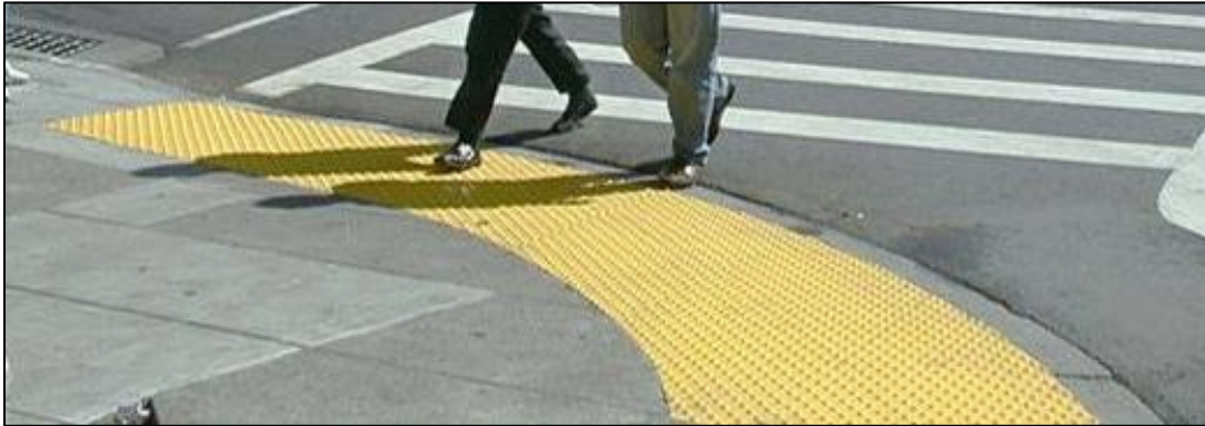
Diagonal blended transition. Note the level transition from the street crossing to the PAR.
