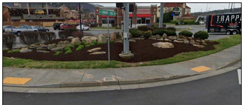
Example of pushbuttons that are not located on an accessible route or which are obstructed.
