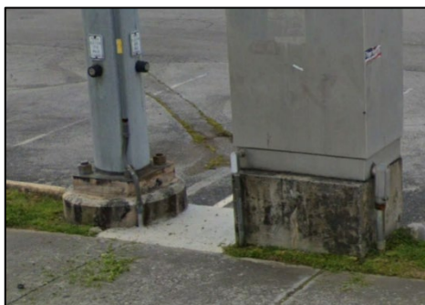
Example of pushbuttons that are not located on an accessible route or which are obstructed.
