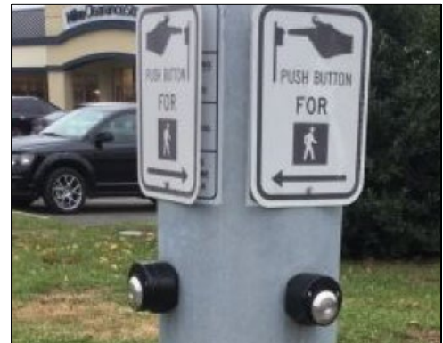
Example of pushbuttons on shared pole.
