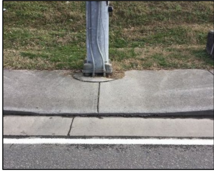
Example of curb ramp with obstruction at the turning space.
