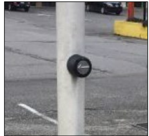
Pushbutton with no signage on pole.
