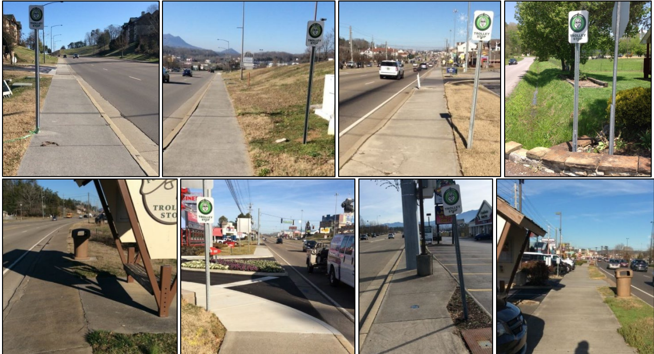
Examples of trolley stops lacking a compliant boarding/alighting area. Many lack the required 5' wide x 8' deep dimensions, non-compliant slopes, have a grass strip between the curb and PAR, or no PAR present.
