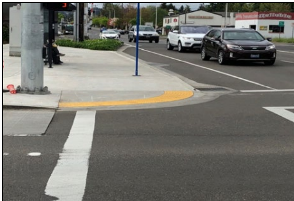
Diagonal blended transition (left) and diagonal perpendicular ramp (right). Both provide access to street crossings of more than one direction and are permitted by PROWAG R207.1 only in certain locations.
