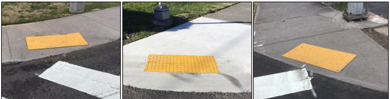
DWs that are oriented poorly and are not 24" depth in entire direction of pedestrian movement.
