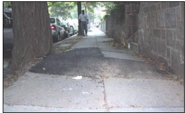
Temporary patching for large displacements
