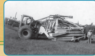
Charles W. Conner, pictured by heavy road equipment used in the construction of the new U.S. Highway 441, the Parkway in Pigeon Forge, circa 1950. Photo courtesy of Bob and Jackie Barnes
